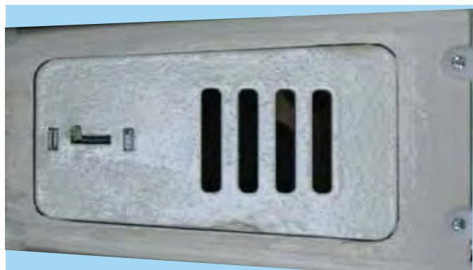
25D - Battery hatch installed
