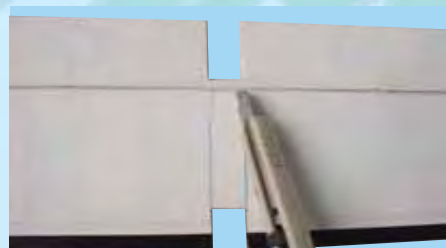
5F- Carefully cut through the covering. Do NOT cut the wood
