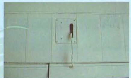
6.3 Aileron control installed
