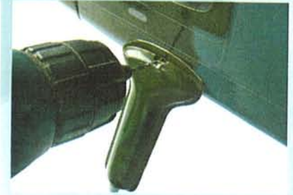
13.4 Pilot drill drill mounting holes with 1/16 (or 1,6 mm) drill-bit
