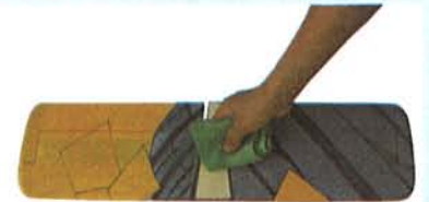
8.2 Cutting inside the lines
