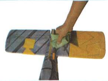
9.3 Wipe off excess epoxy
