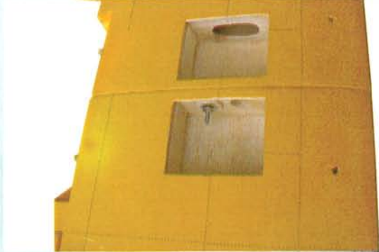
1.5 Use wing bolt clam set to hold the both wing panels together
