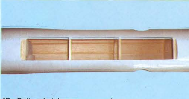
1B - Bottom hatch cover removed
