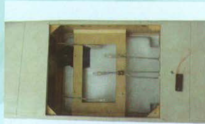
1.1 Removed hatch cover
