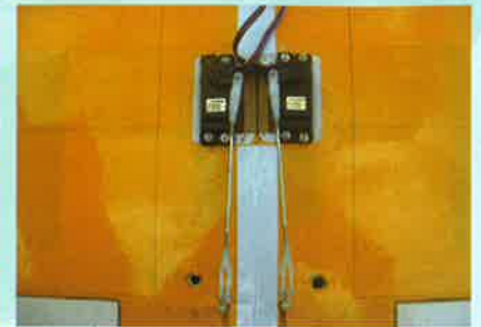
8.3 Aileron control installed
