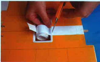
4.1 Apply tape over the joint, starting here
